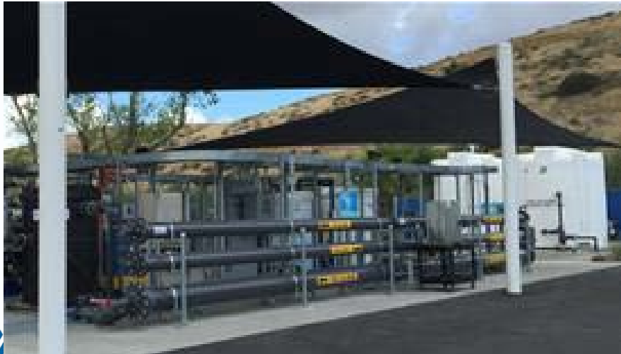
Padre Dam MWD's Advanced Water Purification Facility Demonstration Project
