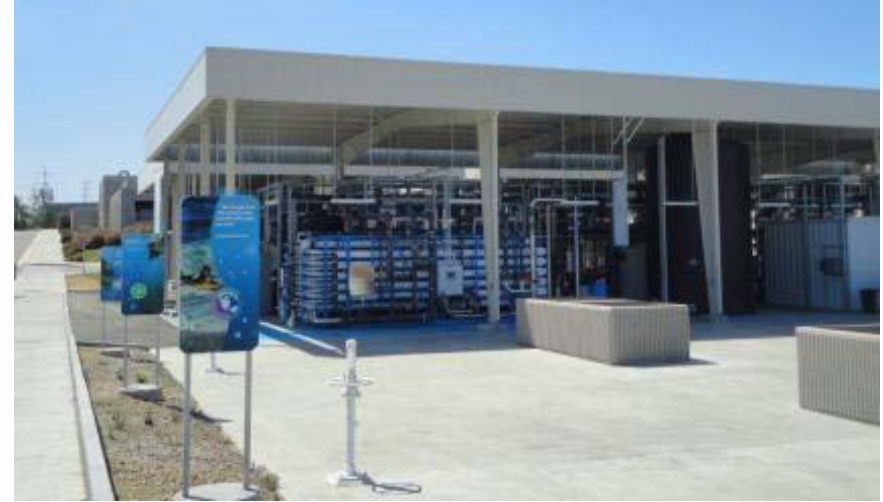
City of San Diego's Pure Water Facility Demonstration Project
